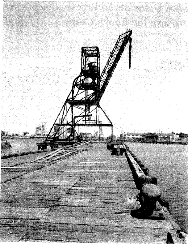
Figure 1 The Copra Crane at Islais Creek
